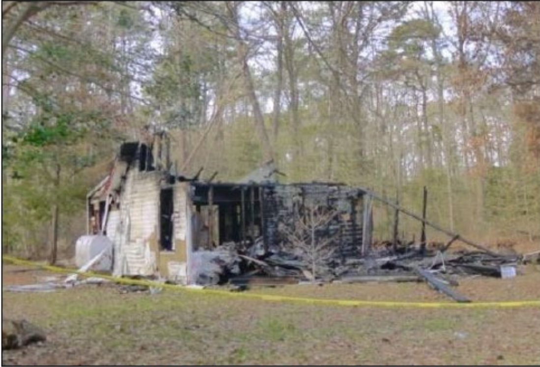
Image #3: The above example image represents damage as the result of a fire.
